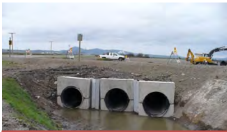
No Name Slough Bypass Culverts
