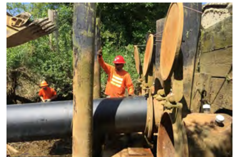
Chilberg Pump Discharge Pipe Lining
