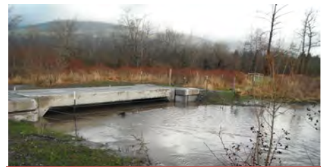
Red Creek Culvert Replacement
