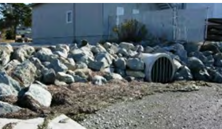
Bay View Padilla Bay Culvert Extension
