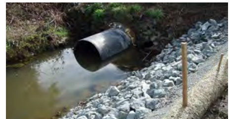
Brown Slough Pipe Lining
