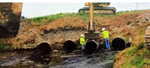
Samish Flood Return Pipe Lining
